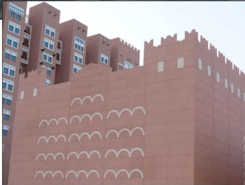
MRS Robotic Parking Building Ibn Battuta Mall, Dubai Exterior Finish: Mineral Life Textured Silicate Paint
